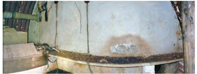
Back wall of the dugout
